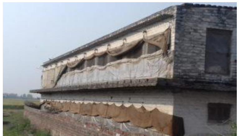
Use of gunny bags for prevention of cold air entering in shed
