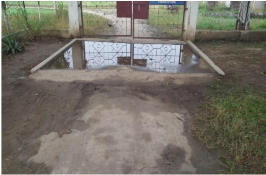
Fig.2. Photograph showing the Vehicle bath for piggery farm
