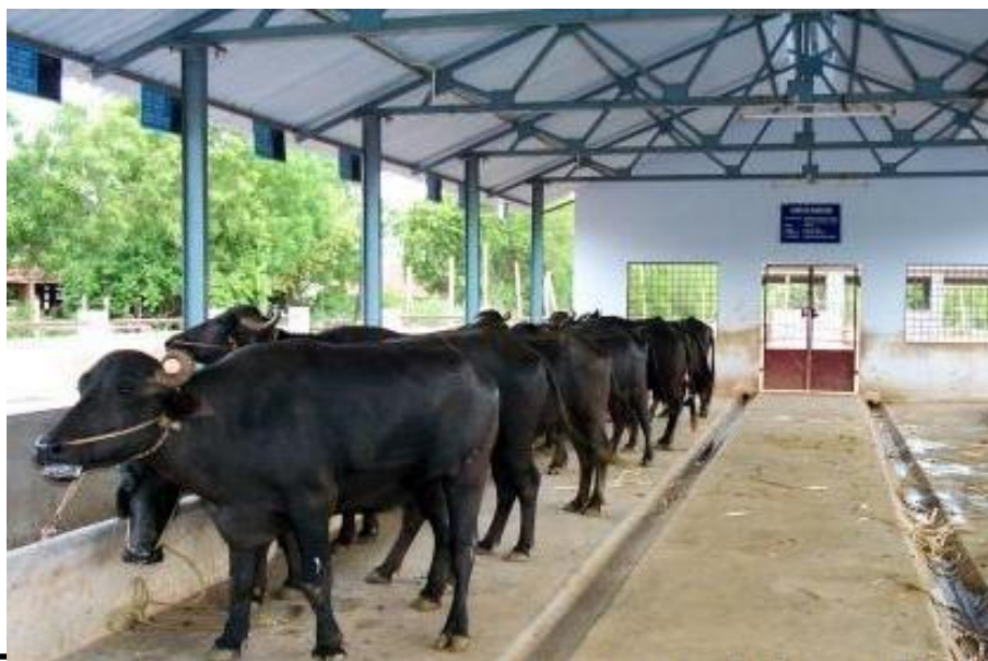
BUFFALO SHED WITH ASBESTOS SHEET ROOFING
